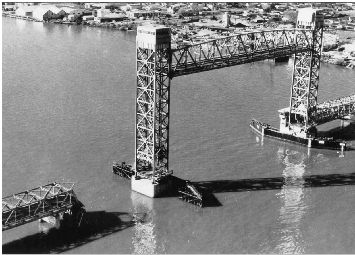
Rio Vista Bridge, January 1967, after Italian freighter Illice took out 100 feet of the bridge structure.
